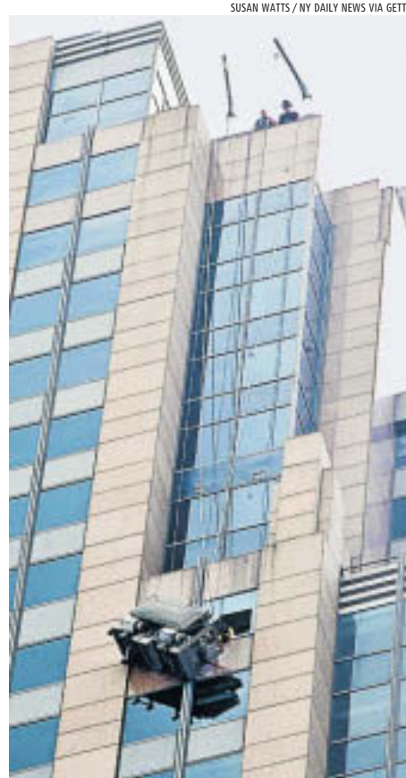
Firemen cut holes through glass to save the window cleaners on a New York skyscraper
